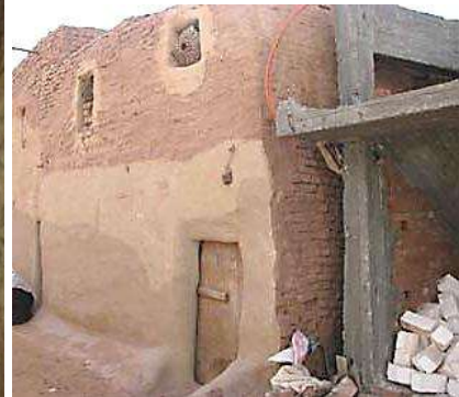
Figure 17: Replacement of mud brick vernacular houses with concrete skeleton ones.
