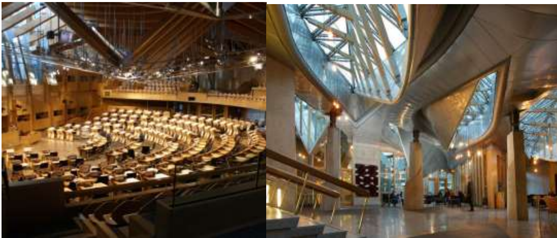
Figure 9: Natural light diffuses into the chamber and is provided by "glass fins" which run down from light spaces in the ceiling. Curved slices have been taken out of the vaults to allow daylight to penetrate down. Source [10]
