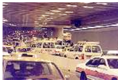
Figure 9 : Tunnel shape causes sound reflections.
