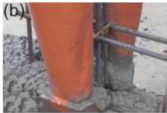
Fig 6: Integrating traditional steel reinforcements with 3D structural concrete printing (1)
