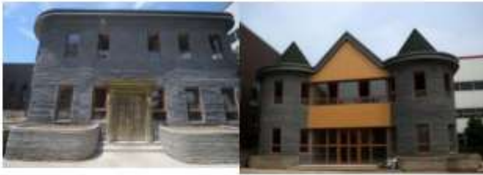
Fig 5: A two-story villa built entirely using 3D printing technology from Huashang Tengda (1)
